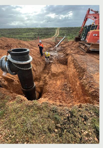
The Inkerman Gas Collection System (GCS) expansion has reached completion, with us successfully installing 59 landfill gas (LFG) extraction wells, spanning over 5 kilometres of flow, lateral and header lines, and a highly efficient condensate management system.
